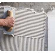
For permanent installation of ceramic, porcelain, vitrified tiles on horizontal masonry surfaces in the interior as well as exterior. It is also used for installing marbles and granites on floors and other horizontal surfaces only.
