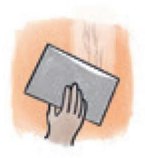
Surface imperfections such as holes, dents, fine cracks are to be filled with crack filler, before painting.
