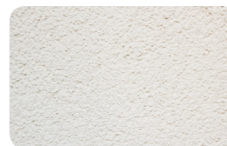
New and existing plasters
