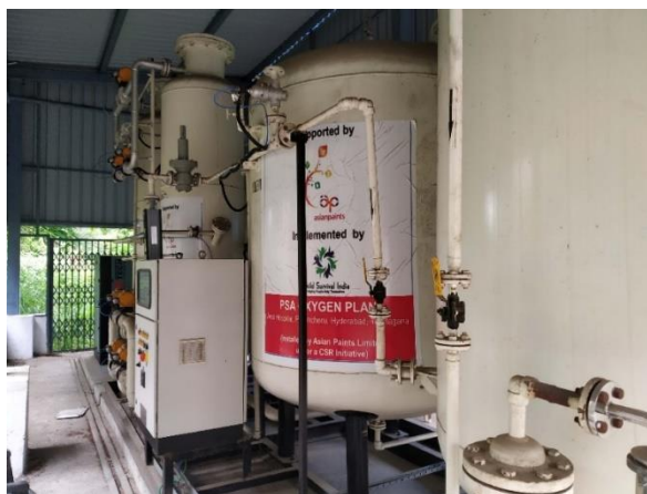
Figure 1.1: Oxygen Plant installed by APL at the Area Hospital
