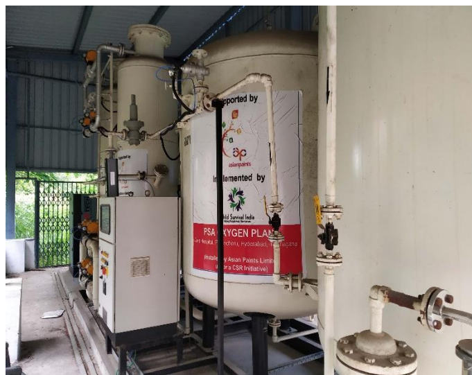
Figure 7.12: Oxygen Plant setup by APL
