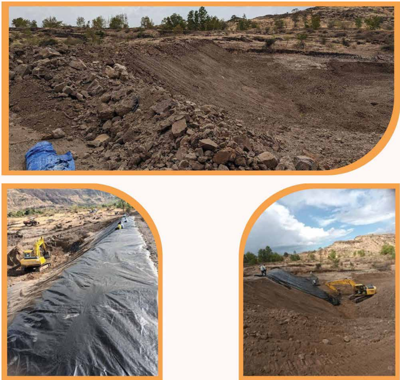
Figure 57 : LDPE sheet being installed over Earthen Nala Bunds
