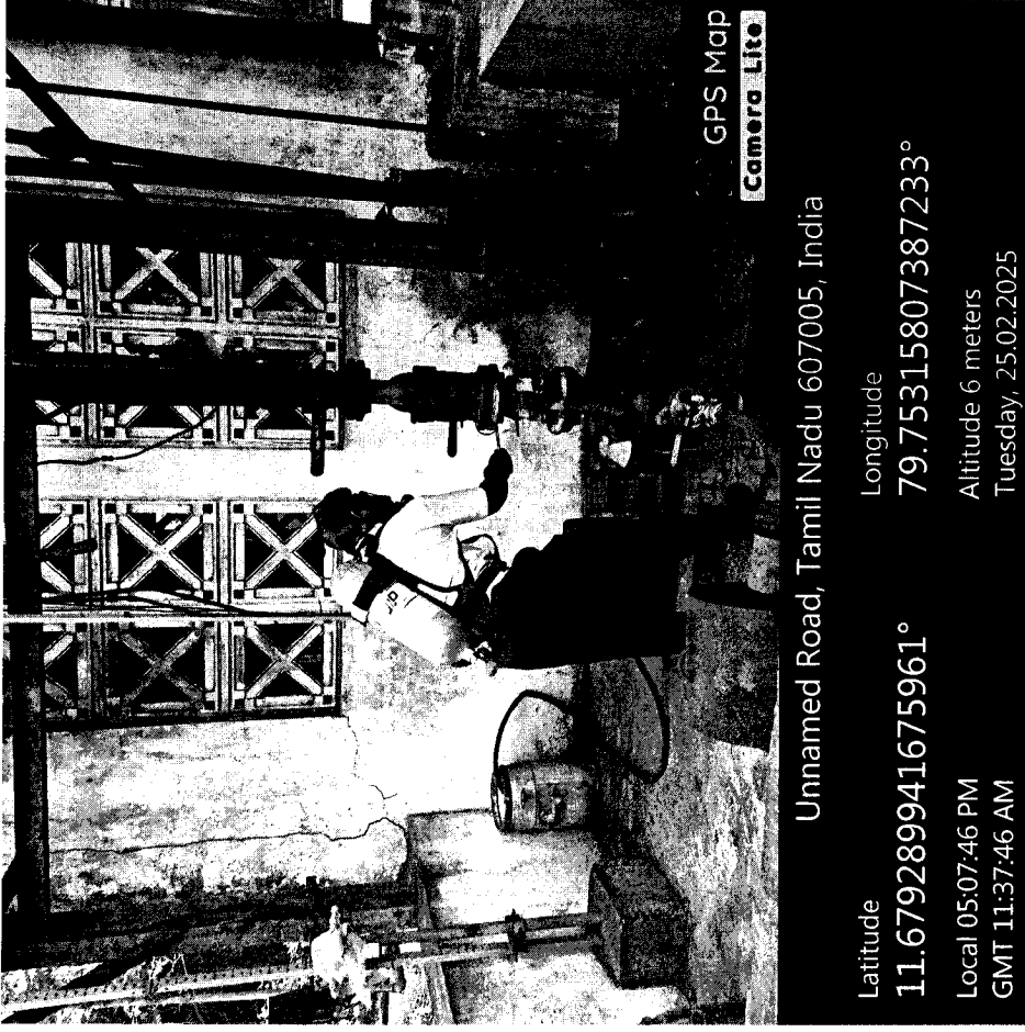
Fitter arresting the Acetaldehyde leak wearing SCBA(Self Contained Breathing Apparatus)
