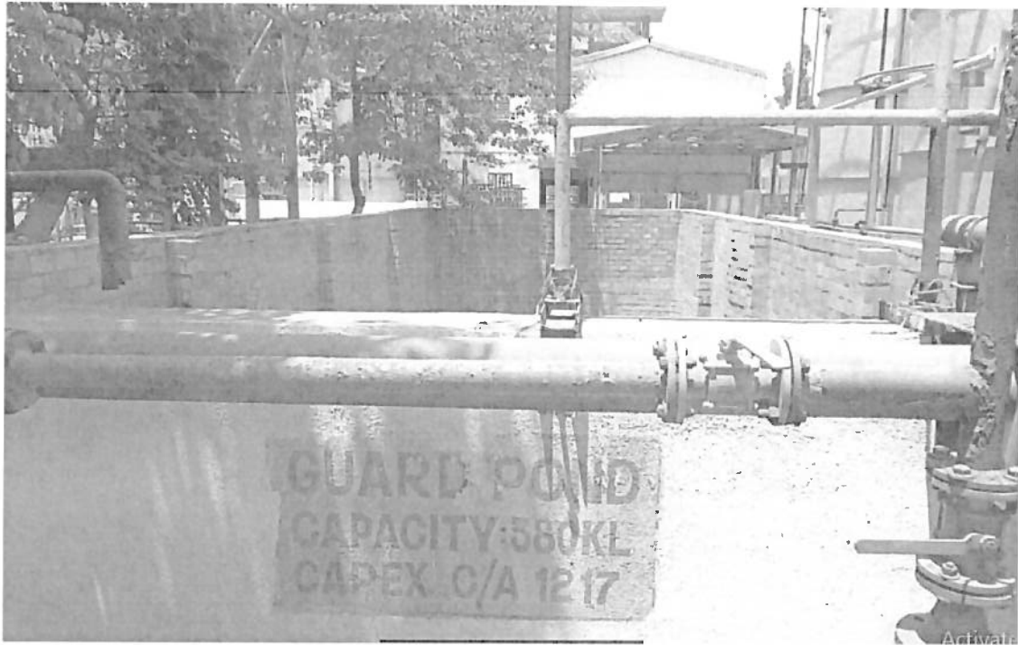
Guard pond of 380 KL capacity
