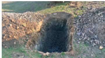
Recharge pits dug in low-lying areas of the field
