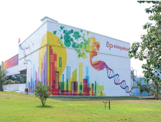
Research & Technology Centre at Turbhe, Navi Mumbai
