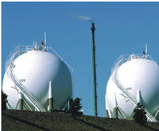
Tanks painted with high performance coatings
