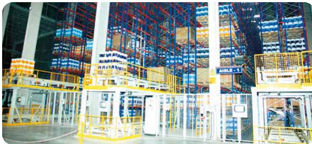
Distribution Centre at the Sriperumbudur plant
