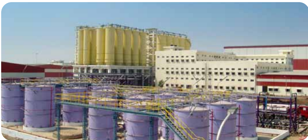
A view of tank farm and silos at the Rohtak plant
