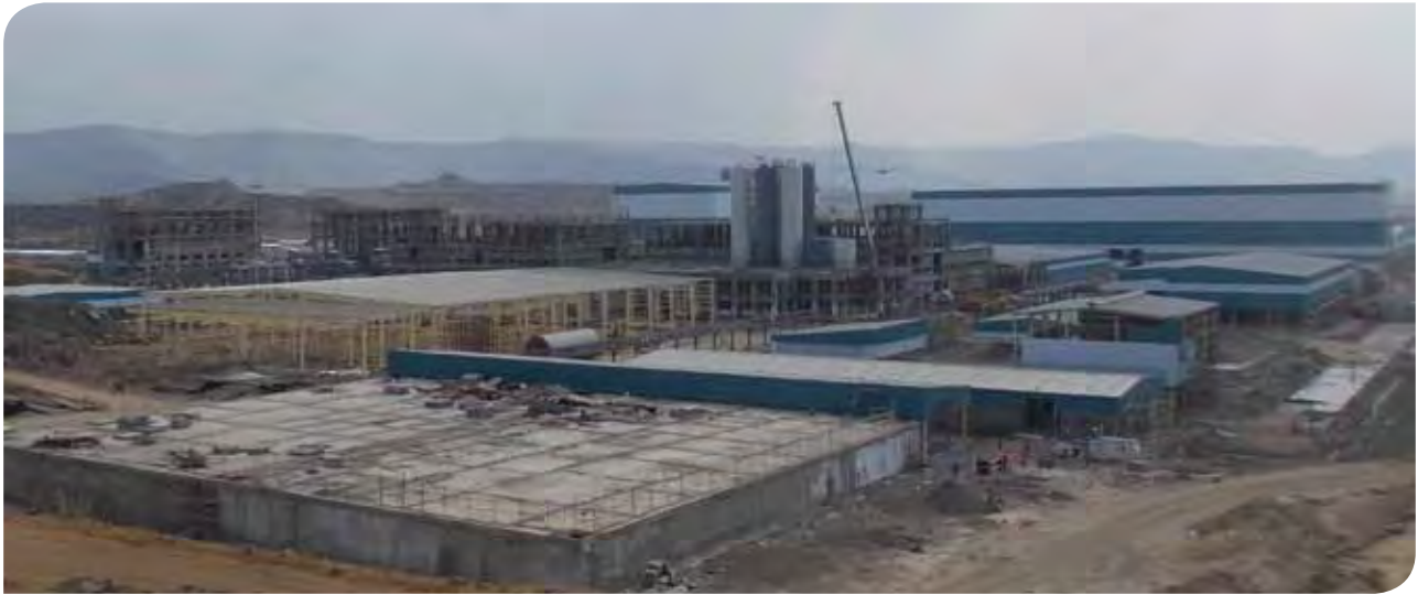
Khandala plant under construction
