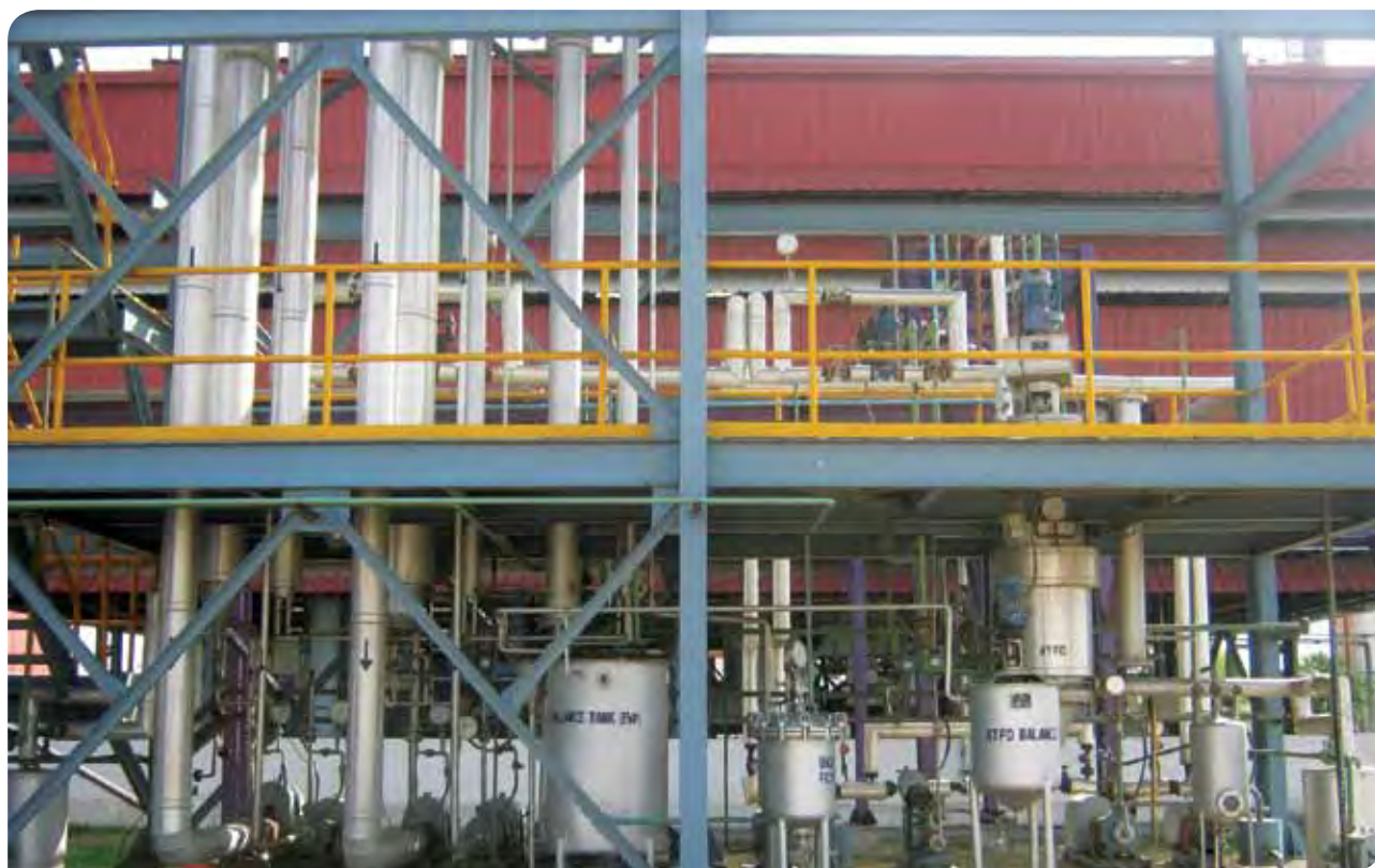
Process unit for Water recovery from Waste-Water installed at Rohtak Plant
