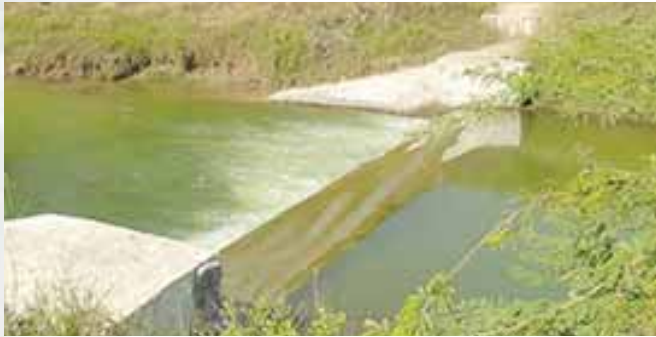
Construction of check-dams
